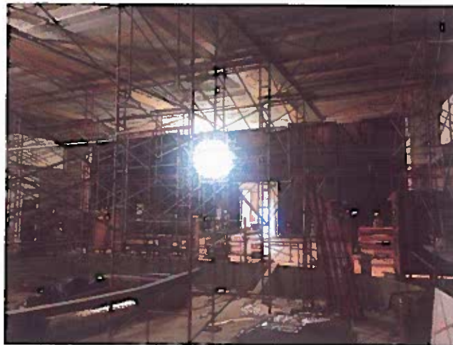
Auditorium - Seating Area
