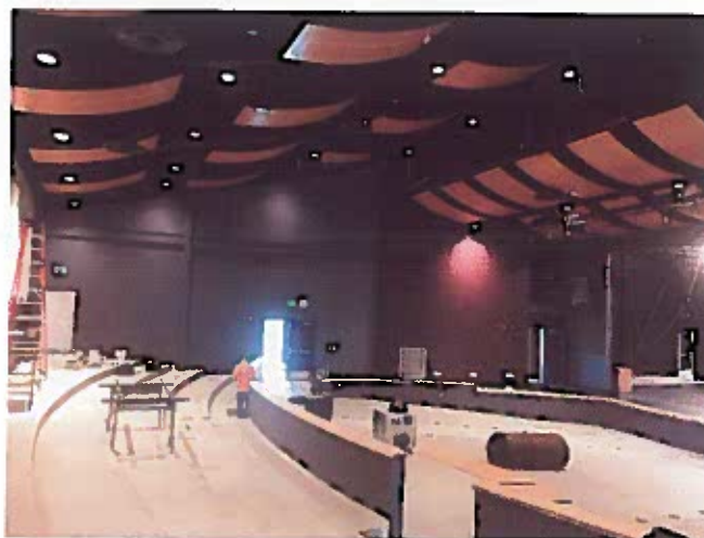
Auditorium - Seating Area
