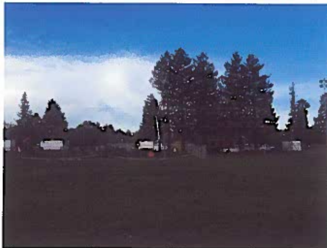
Creekside Trail/Track & Field – Tree Removal
