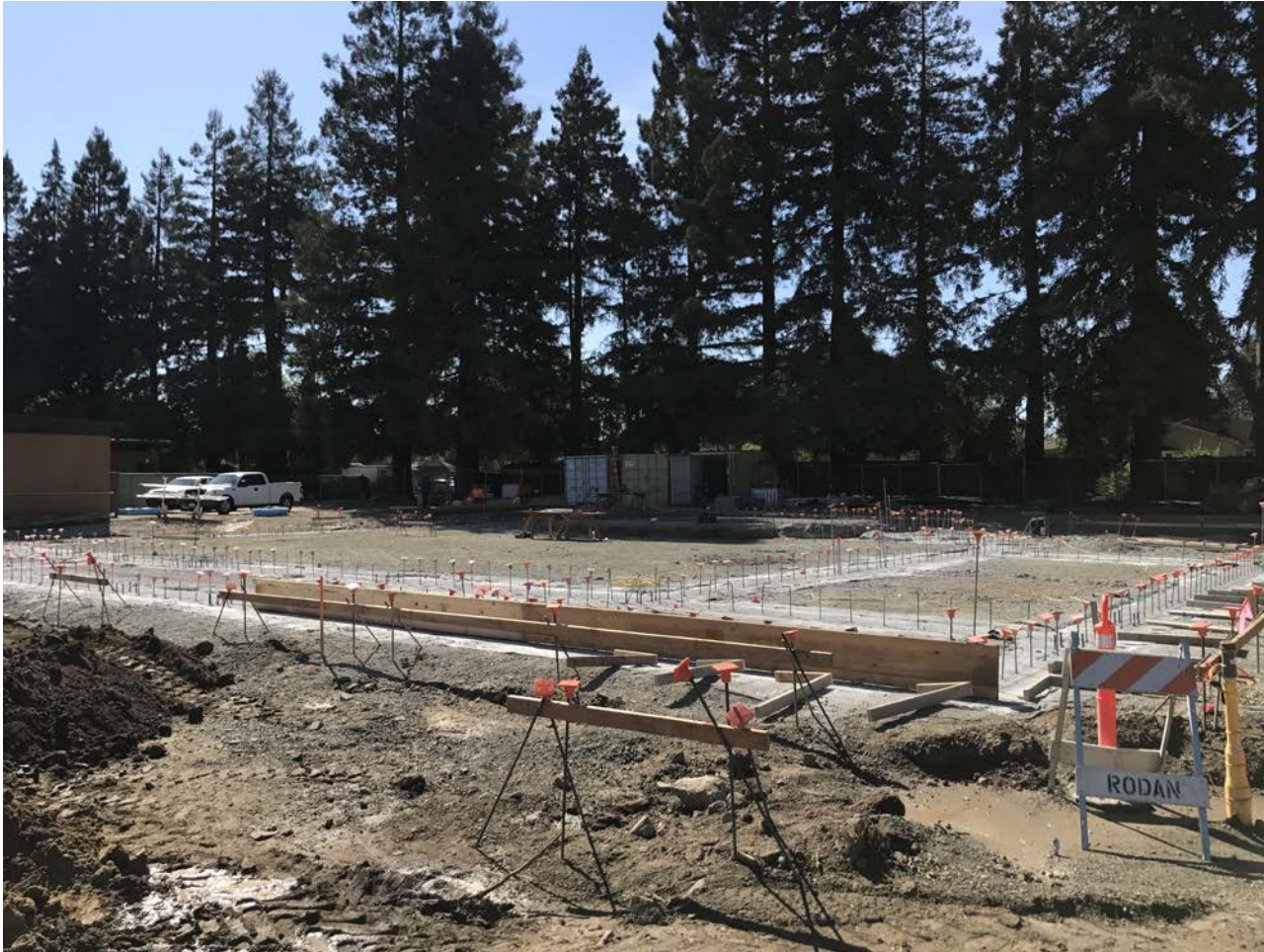
Landels MUR New Construction
