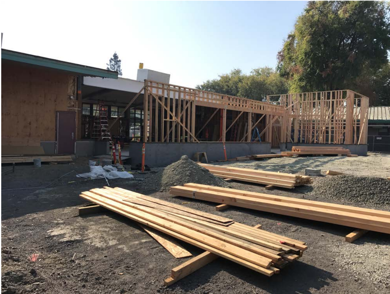
Monta Loma MUR New Construction
